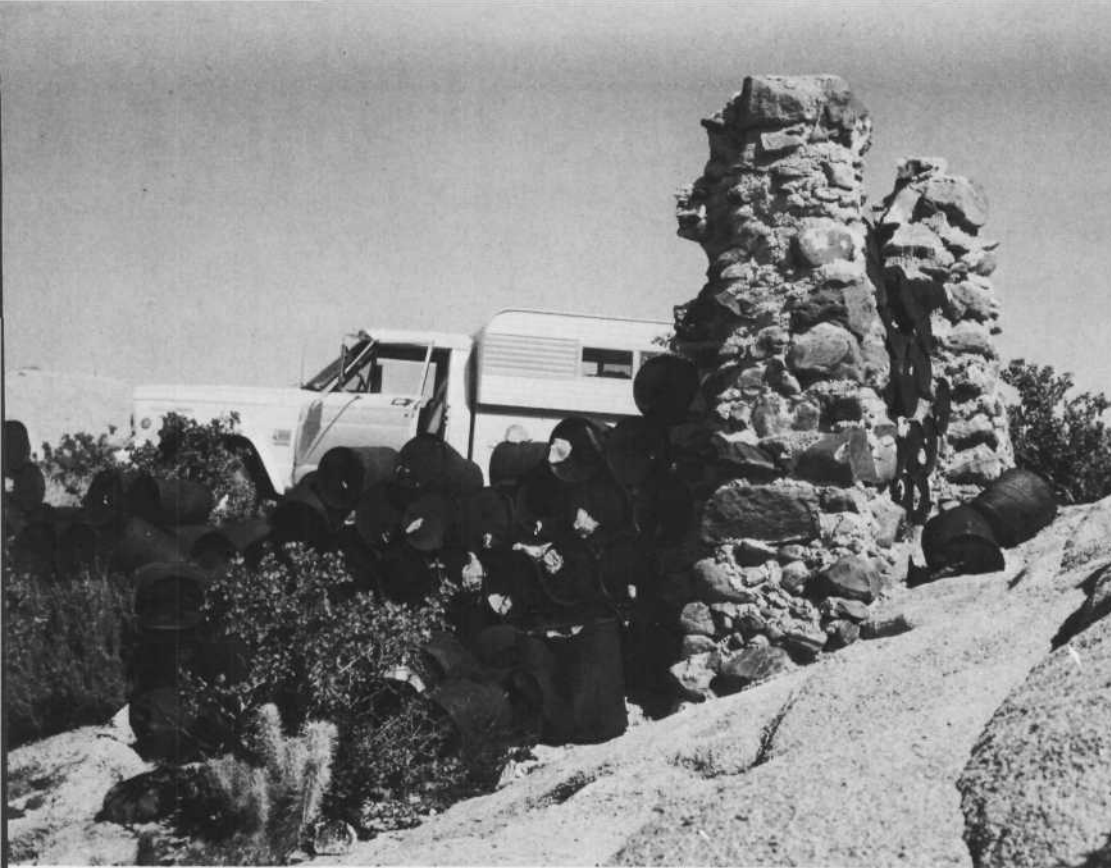
Empty explosive cans were used in the walls of this house at the upper camp.
